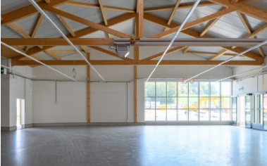
Exposed timbers inside Generous sales rooms
